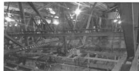
Figure 9 – Auditorium roof space showing modified transverse truss at lighting bridge
