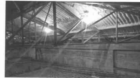
Figure 4 – Stage house roof structure (a lack of diaphragm bracing is evident)
