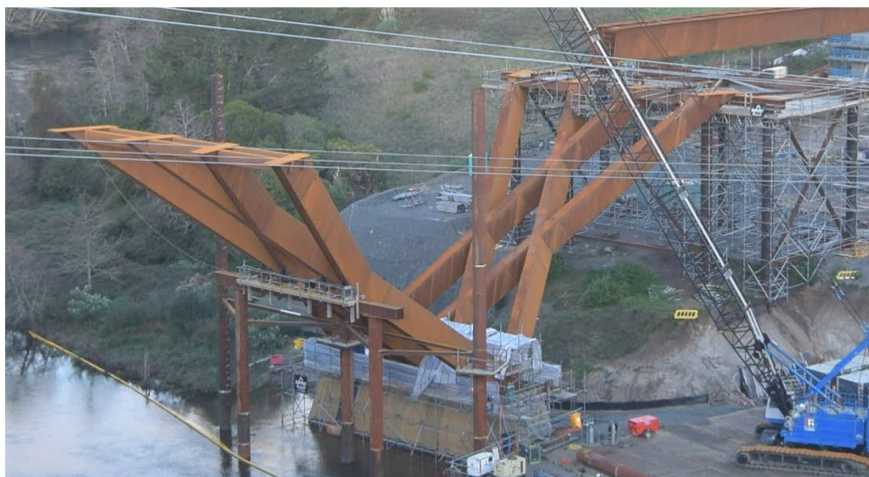
Figure 9: Central Y-shaped pier lattices
