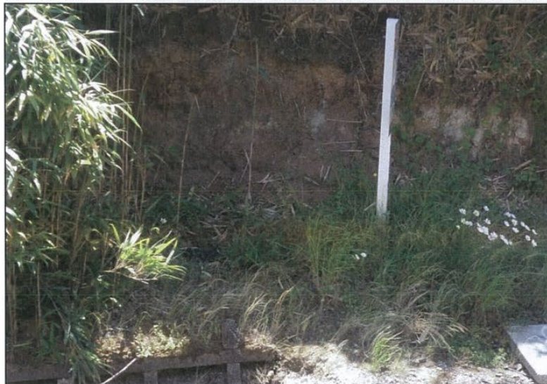
FIGURE 21 LOW LEVEL RAILWAY EMBANKMENT NEAR SONNING CAR PARK (Note: bamboo and soil profile with shallow top soil and no topsoil-subsoil interface)
