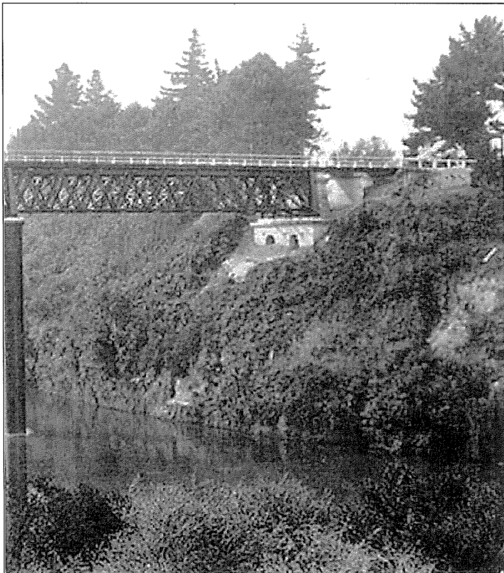
FIGURE 9 EASTERN ABUTMENT OF HAMILTON RAILWAY BRIDGE CIRCA 1910; VIEW NORTH EAST (Hamilton City Library #11248) (Note: terraces on the south side, probably created to stabilise the slope. There is also evidence of earthworks on the north side of the bridge.)
