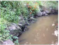
Figure 10: Toe protection at MGK\_Main\_5.
