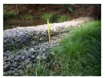
Figure 124: Carbourne Wetlands fish barrier.
