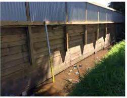
Figure 26: Timber bank lining along property at MGK\_C\_Fork1\_2.
