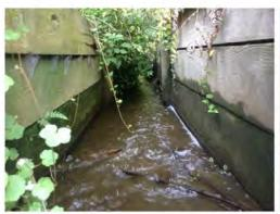
Figure 25: Bank lining extending 40 m at MGK\_C\_Fork1\_2.
