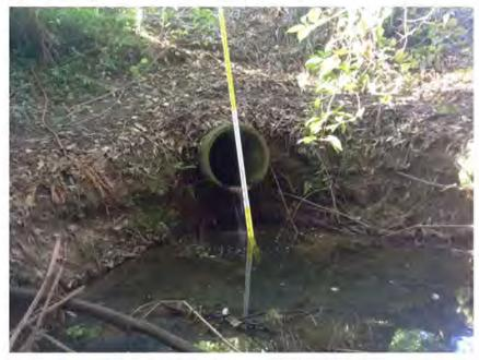
Figure 120: Perched culvert presenting a fish barrier in low flows.
