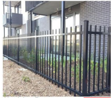
Aluminium Fence 1.2m high aluminium post and vertical bar infill fence
