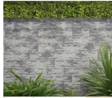
Keystone Retaining Wall Height varies 0 > 700mm
