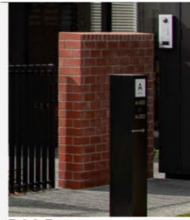
Brick Fence 1.8m high double brick fence
