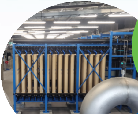
Membrane Plant Filter Racks
