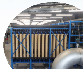
Membrane Plant Filter Racks
