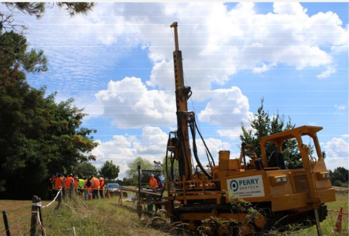
Geotechnical testing of the bridge site
