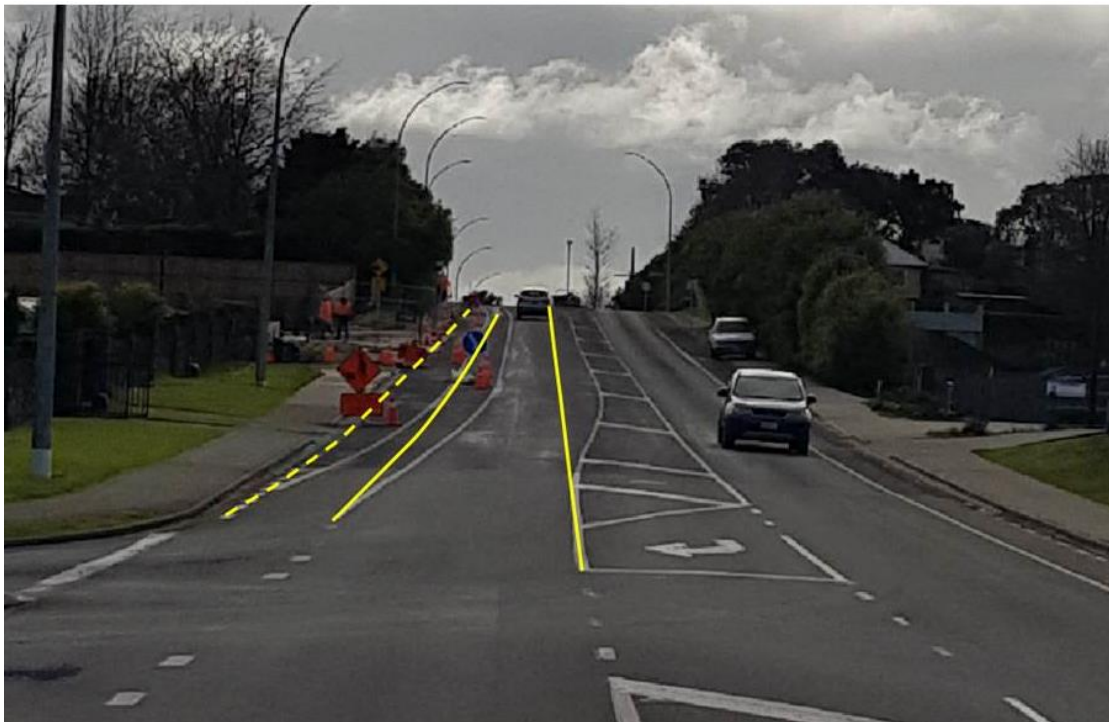
Figure 2: Looking north along Horsham Downs Road towards North City Road – proposed cycle lane and central median for right turn bay into new development.
