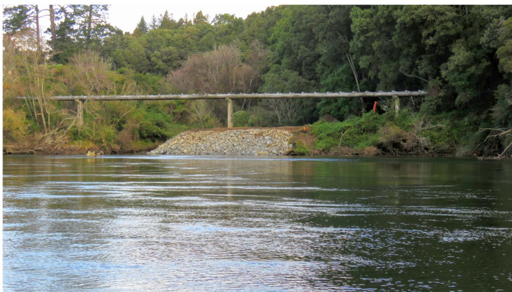
Western Bulk Watermain Pier B scour remediation.
