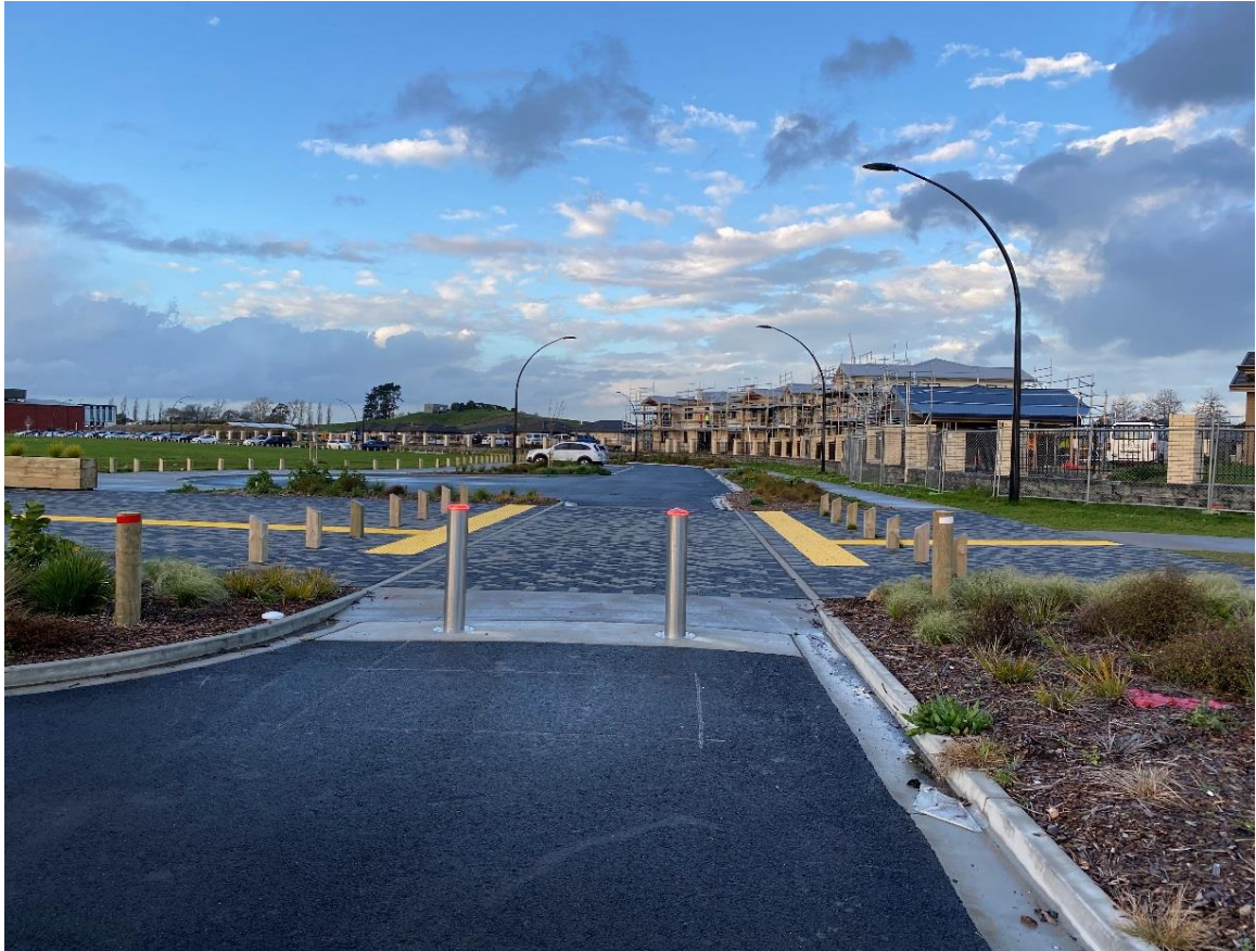
Figure 2: Raised pedestrian platform with bollards raised.
