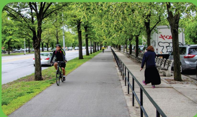
Wide separated bike path with physical barrier
