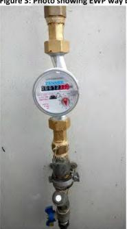
Figure 3: Photo showing EWP way bay water meter
