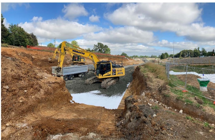
Excavation to create northern bridge abutment on the Hamilton Gardens side of the river – February 2021
