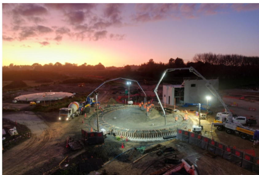
1 Transfer pump station wastewater tank base slab pour - pump station building in background – 2023.
