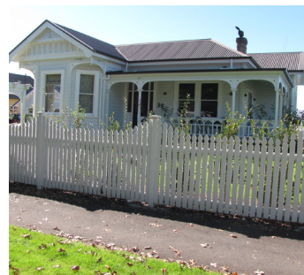
Return bay added and connected by a return verandah
