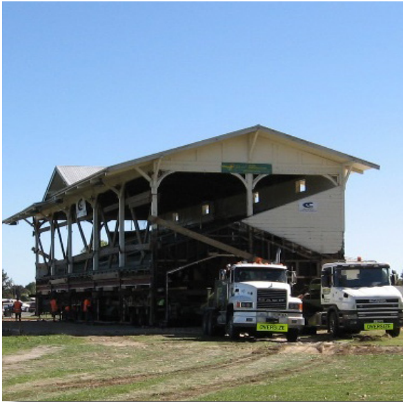
Above: Claudelands Grandstand being relocated on the same site
