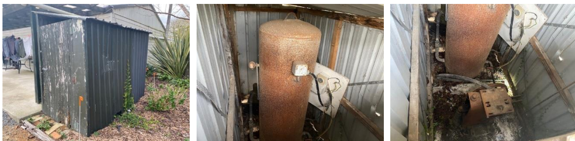
Old bore and pressure tank (not operational)
