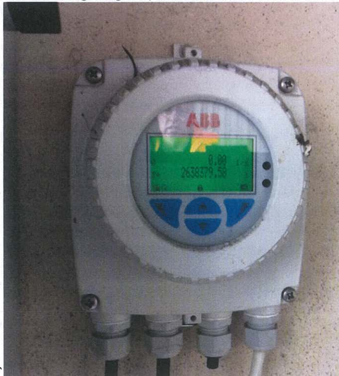
Figure 2: Photo showing the waste flow meter reader at Kiwi Rail
