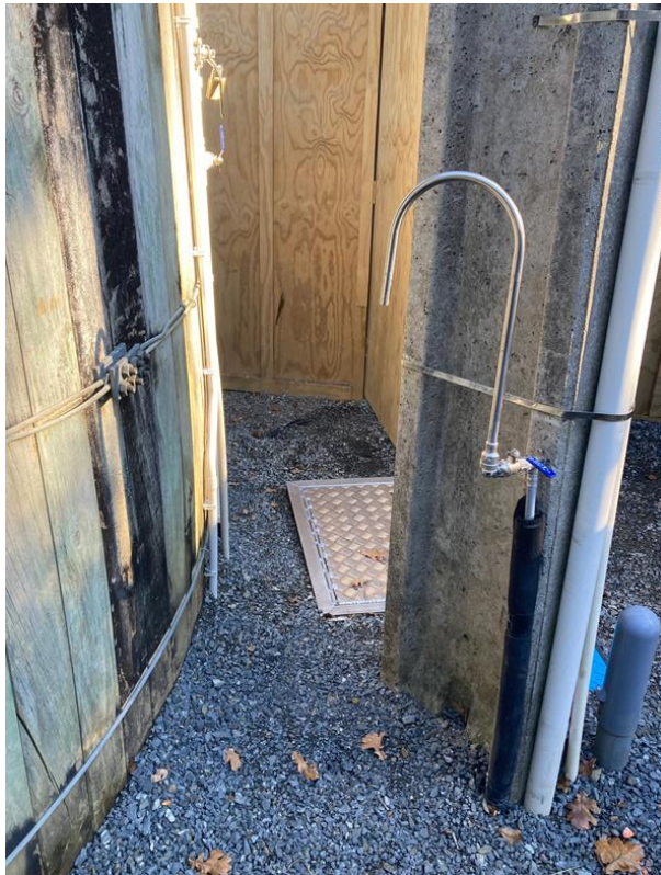
e) Reservoir tap (treated water) – replaced
