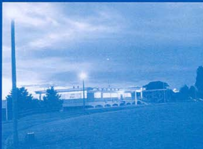
Wastewater Treatment Plant, Pukete Road, Hamilton.
