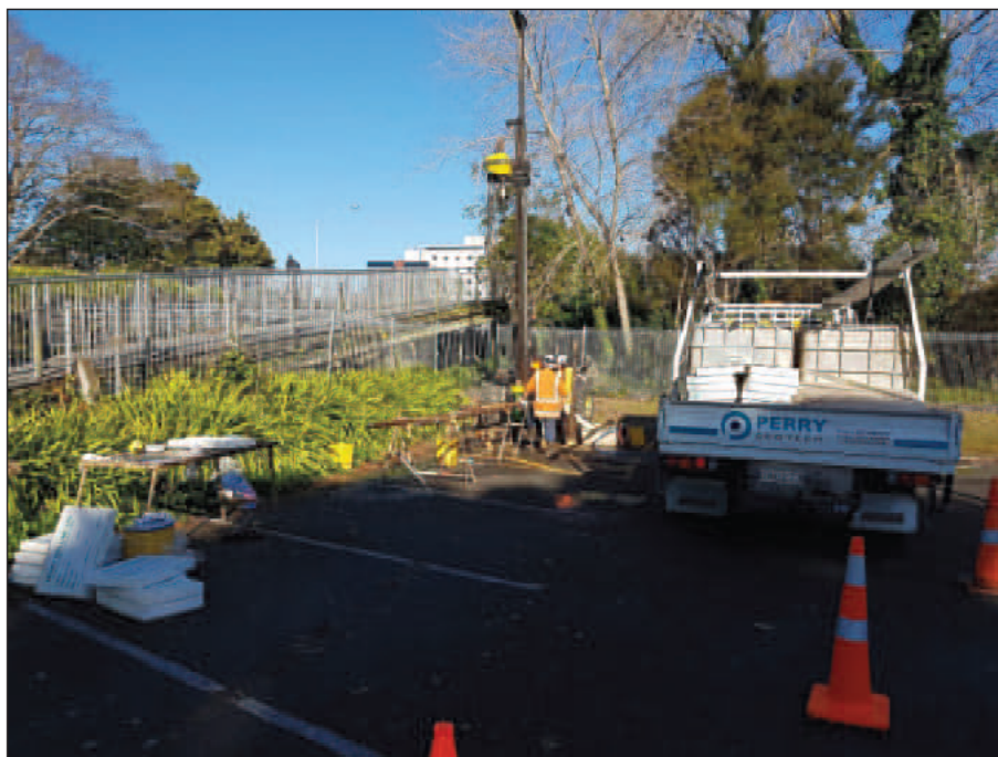
Photo BH1.9 Site looking westward towards Claudelands Bridge
