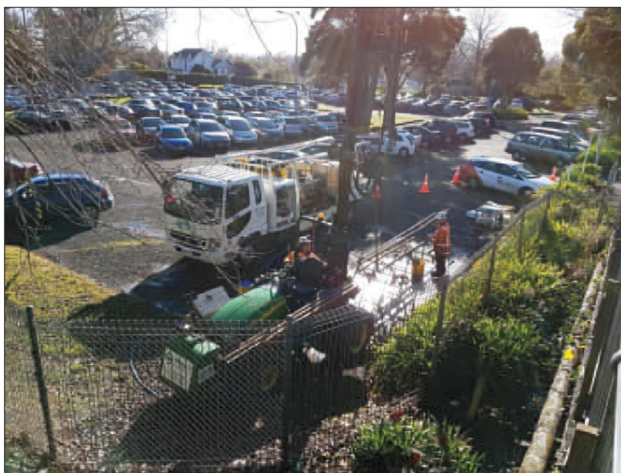
Photo BH1.10 Site view from footbridge over carpark
