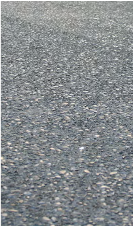
INSITU CONCRETE Exposed aggregate finish.
