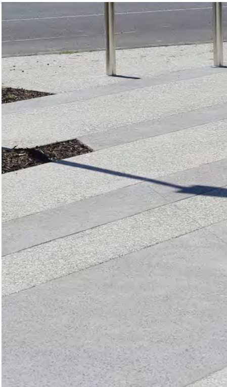
INSITU CONCRETE Exposed aggregate finish. Firth 'Mountain Burst' and 'Manorfield' aggregate. Wintec Rotokauri Campus
