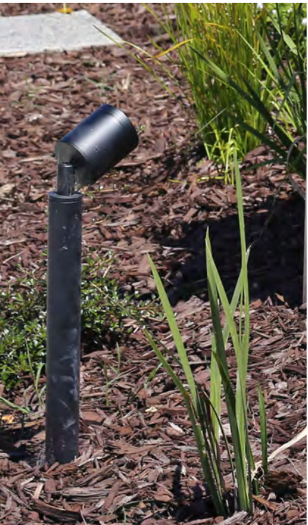
LIGHTING Tree spot lights with a black powder-coated finish. Wintec Rotokauri Campus
