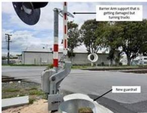
Fig. One: Rail barrier arm being hit by trucks
