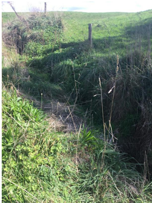
Image 13: Farm drain with intermittent water flow along watercourse five.
