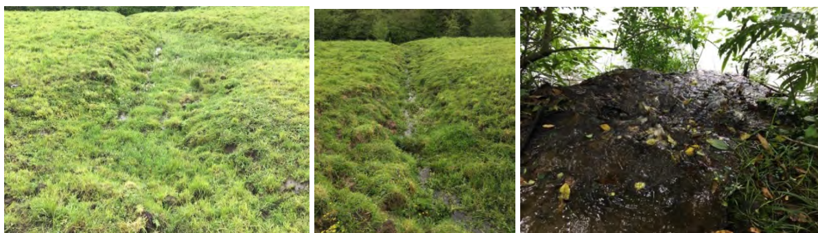
Plate 1: Watercourse 5 channel (left and middle) and perched outfall to the River (right).
