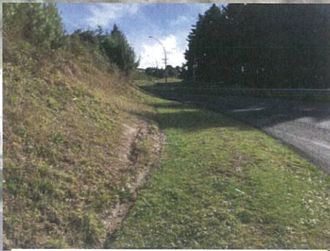
PHOTO 1. BATTER SLOPE WHERE EARTHWORKS REQUIRED FOR ROAD WIDENING AND VISIBILITY.
