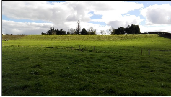
Photo 1: Example of terrace with over steepened back slope.
