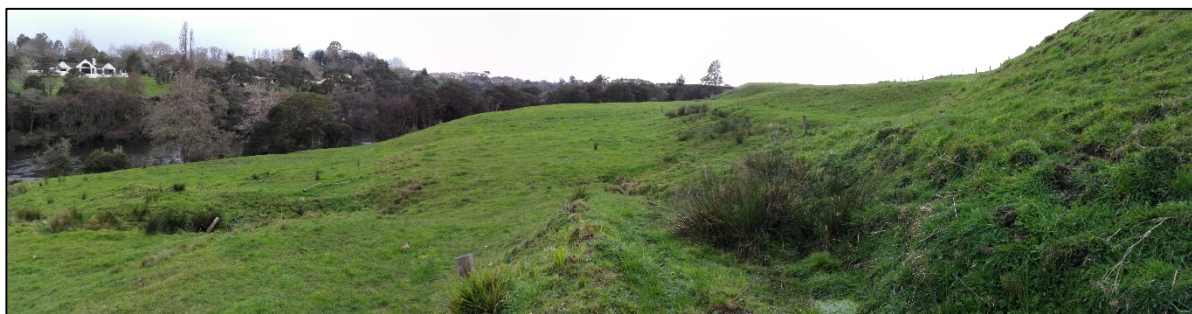
Photo 5: View south along slope terraces, landslide debris and swampy ground adjacent to the Waikato River in the central to northern portion of the site.
