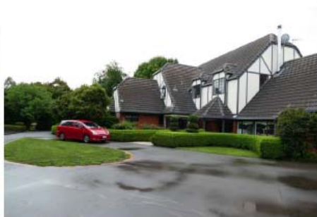
ABOVE FIG. 2-6b: The existing dwelling.
